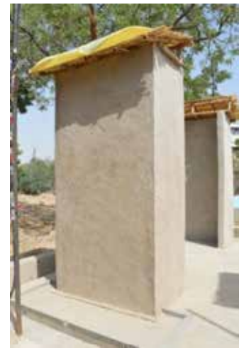
Figure 6. Wall to be tested
