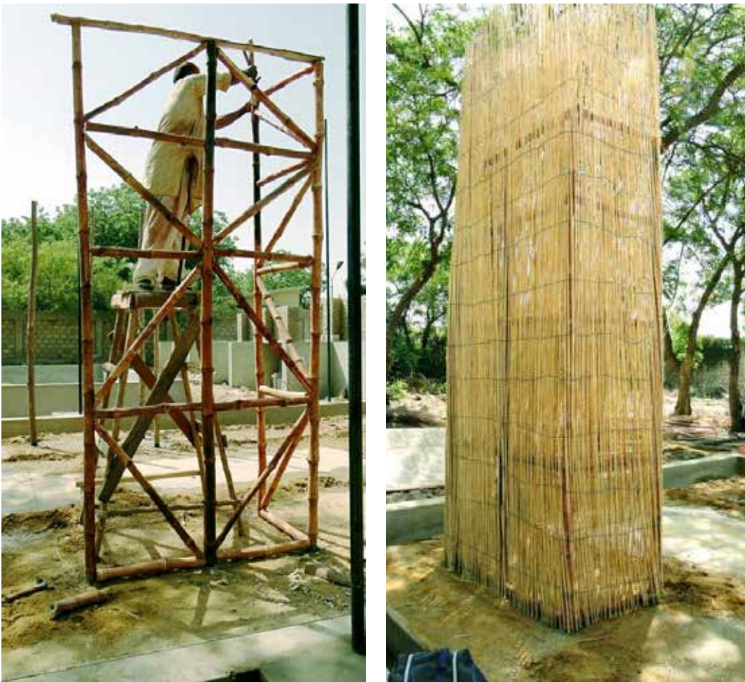
Figure 4 Loh-kat panel at testing facility made from bamboo frame and chicks matting. The next step is to apply plaster to the chicks matting. Note that the bamboo frame requires lots of diagonal bracing in order to make it stable. With many loh-kat shelters recorded as visibly leaning over it is most likely due to insufficient bracing.
